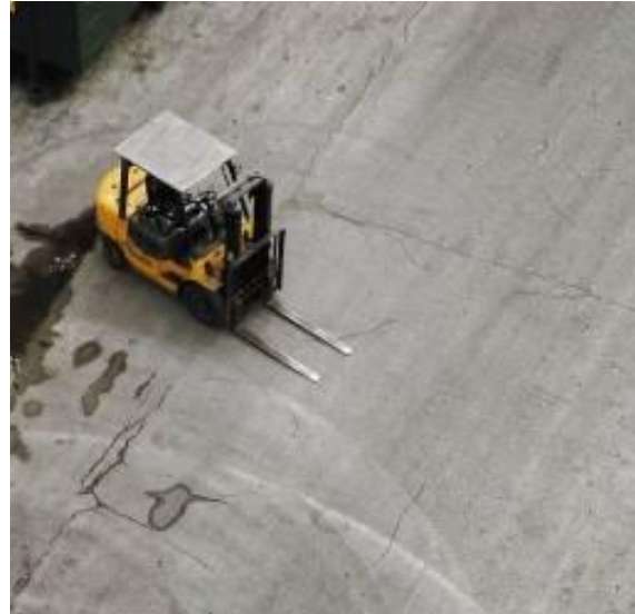
MATERIAL HANDLING/AERIAL LIFT
